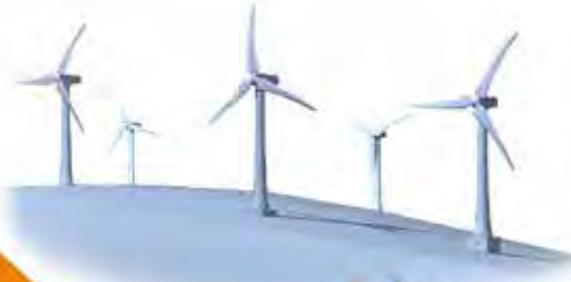
Wind power plant
